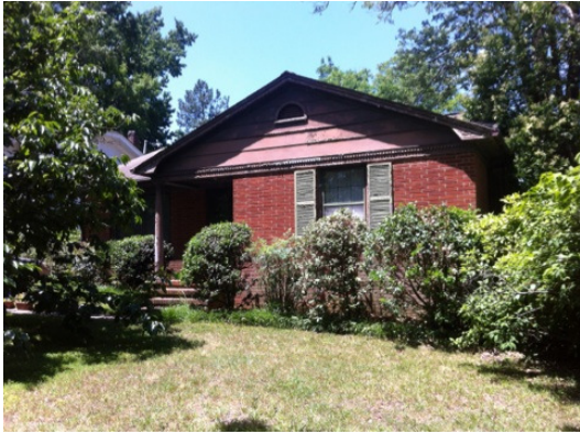
South end of the house
